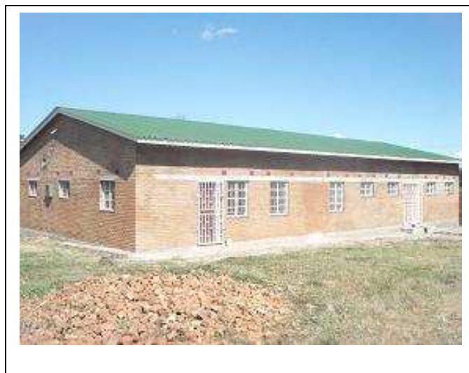
Part of the factory that Zikometso is constructing with the ADF grant
