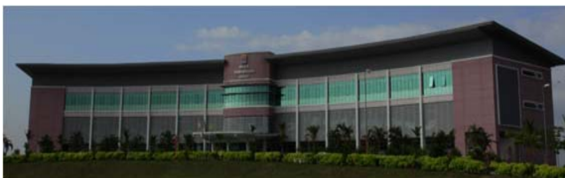
Figure 6 Sepang Municipal Council building
