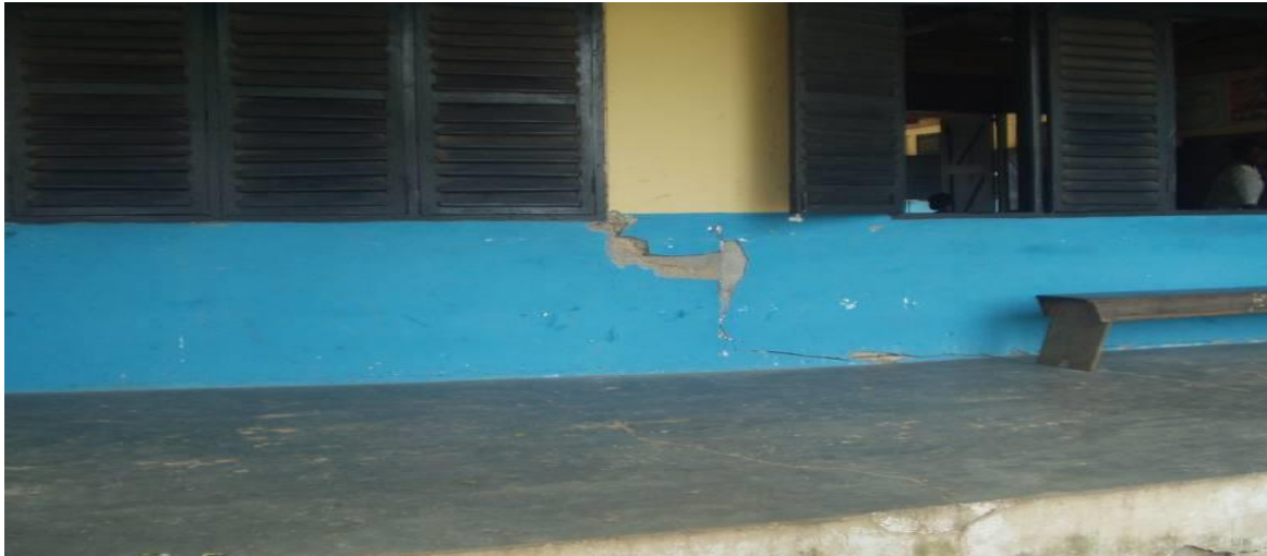
Figure 2. Cracks on the UMAT Nursery School Block
