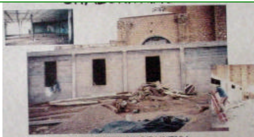
Construction of a Public Library US$267,800
