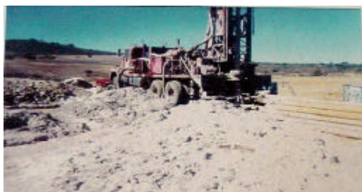
Perforation of a Well for Drinking Water US$359,790
