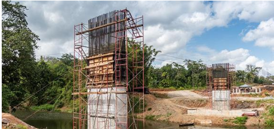
Figure 2 Construction of bridges on El Rama – Kukra Hill Highway Project
