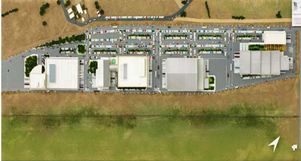
Figure 5: The warehouses (Source: www.aia.gr , same processing)
