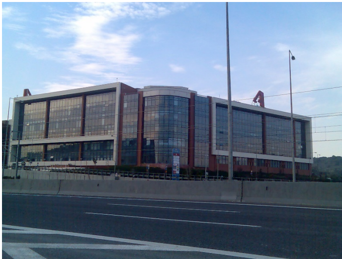
Figure 12: The building of the offices of Alpha on the Attiki Odos (Source: www.google.com )
