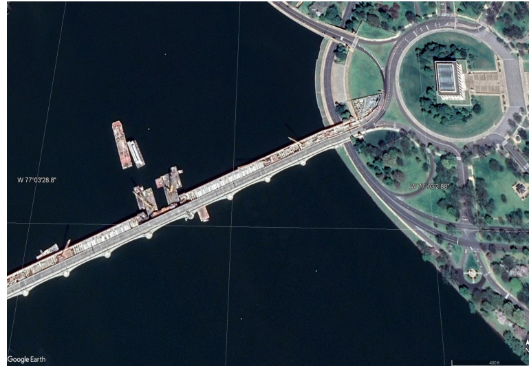
(b) Memorial Bridge, DC/VA Border, March 2020
