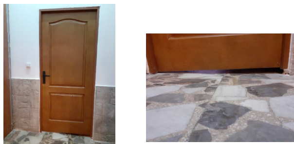
Fig 10. The warehouse entrance door
