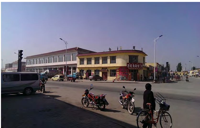
Photograph 24 – Gongtian village, Xixiaozhao County in western Urat Front Banner is a part of the southern transportation route of the Bayannur (G. T. Cirella, 3 October 2013).
