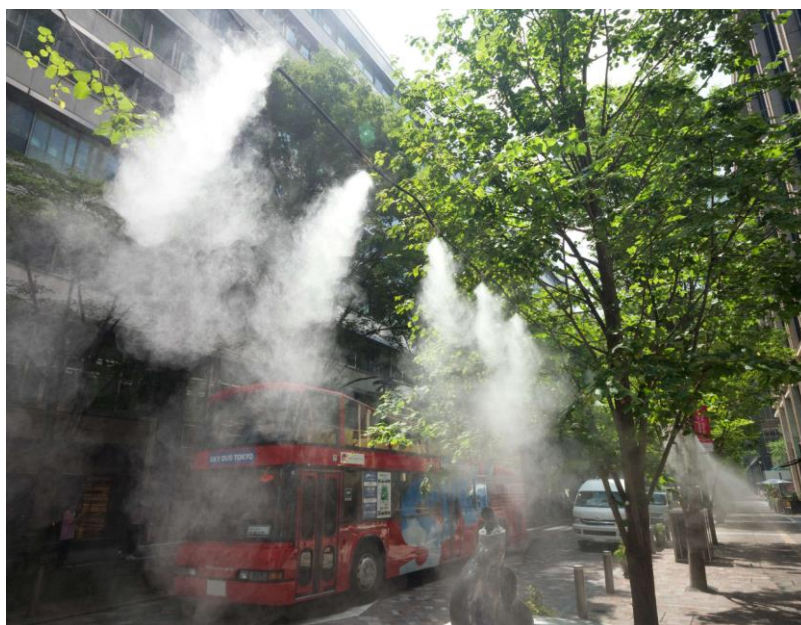
Figure 38. Example of an outdoor misting system to reduce temperature from Marunouchi, Tokyo.
