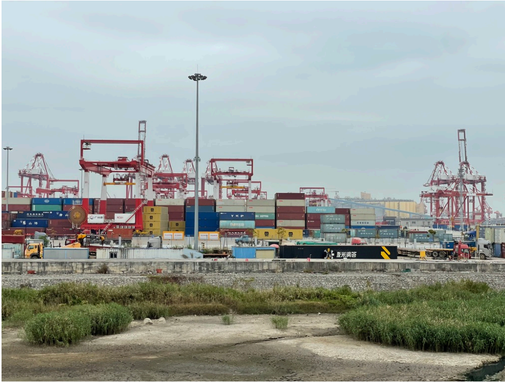
Fig. 2 IGV at Nansha Phase 4 Terminal
