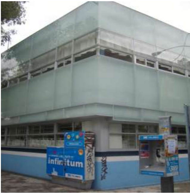
Building that housed Aereofoto in the 1960s (Obrero Mundial # 338, Col. Narvarte). The IBM1130 was located in the second floor. September 2009
