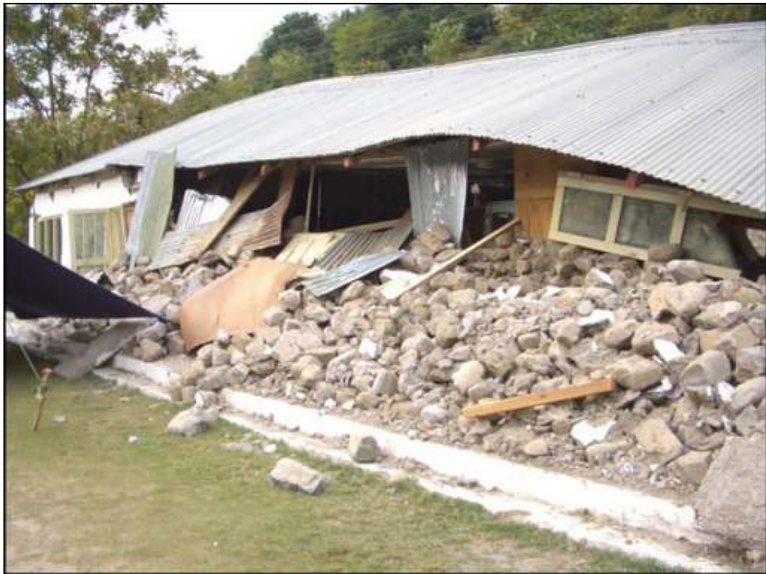
Figure 7: Collapsed Stone Masonry Building
