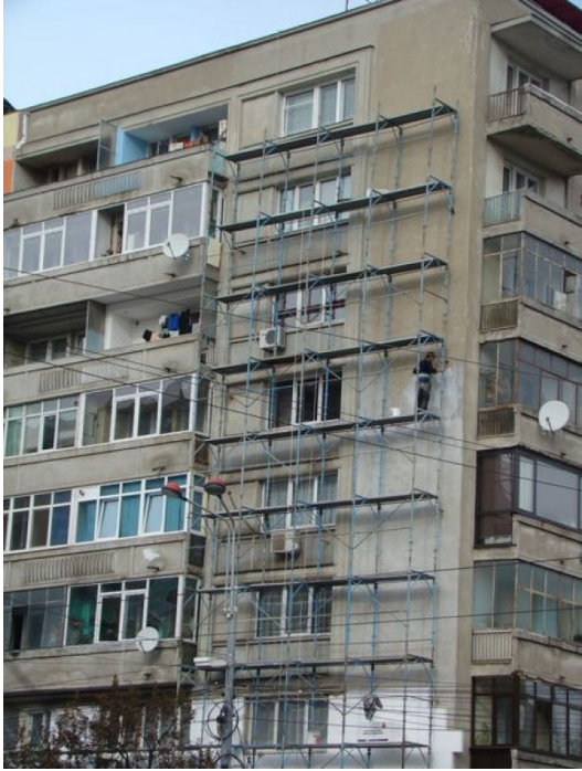
Before thermal rehabilitation- the construction works begin
