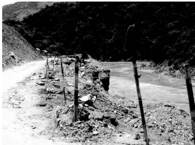
Route No. 7A in Ky Son suffered erosion by the flash flood at Nam Mo River in July 2011.
