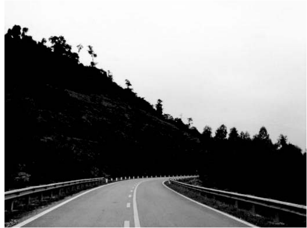
Route No. 12A (AH131) shortcut in Ky Anh District
