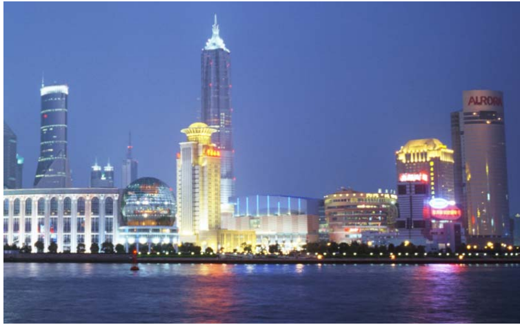
New Pudong District in Shanghai, by the Huangpu River, is home to the Lujiazui financial district.
