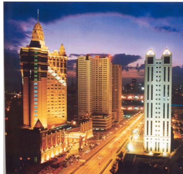
Qingnian Street at night, Shenyang, Liaoning Province
