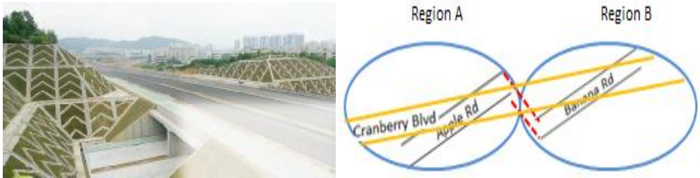
Figure1. Broken-end road (left, source: www.sznsnews.com )
