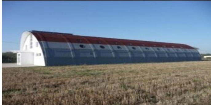
Fig. 1. Prefabricated hall made from ferrocement sandwich elements
