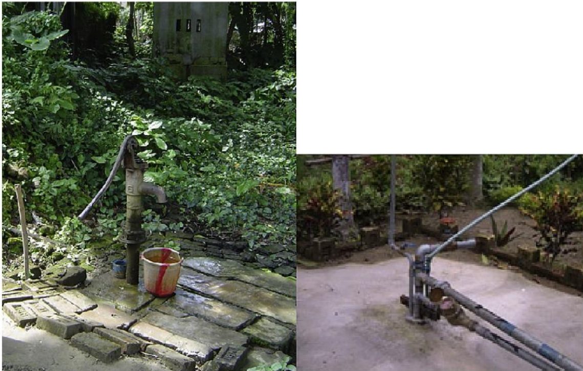
Fig. 4. A view of the site before and after installation of the treatment plant.
