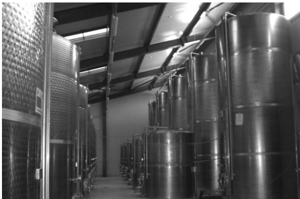
Fig. 8 – Vinification section (equipments for wine storing)
