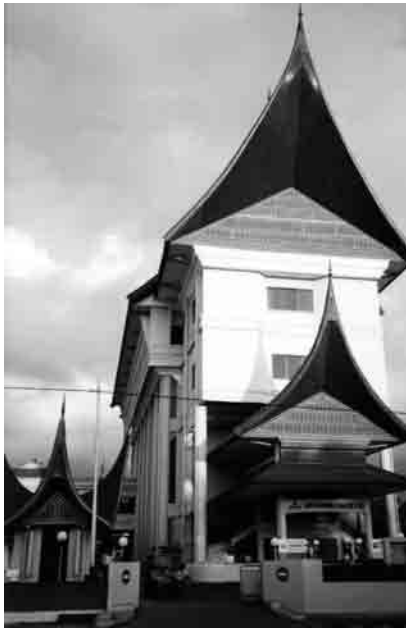
Figure 5: Bank Building, Padang, West Sumatra
