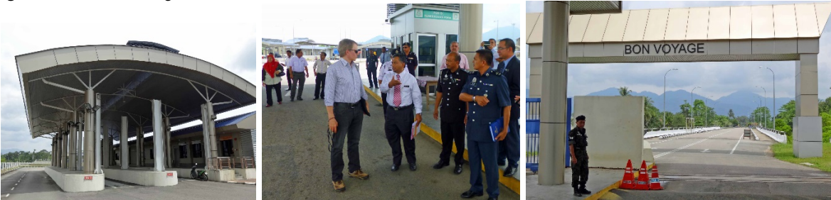
Figure 8.12: Bukit Bunga New ICQS Facilities
