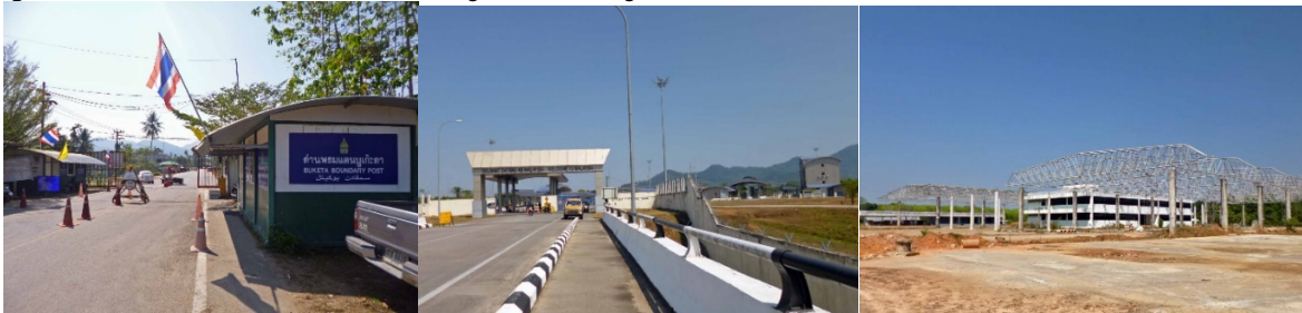
Figure 8.12: Ban Buketa Border Crossing with Existing Facilities and Those under Construction
