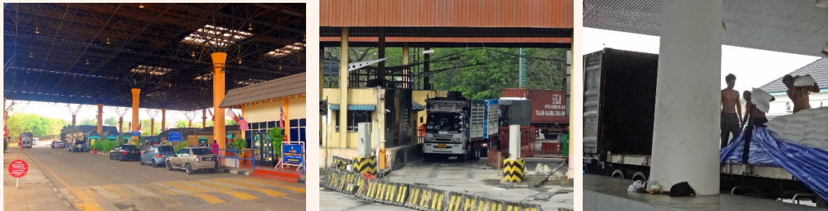
Figure 6.9: Existing Bukit Kayu Hitam ICQS Complex
