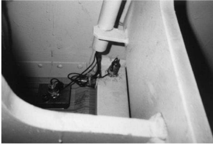
Fig. 4 Core and frame accelerometers [6].
