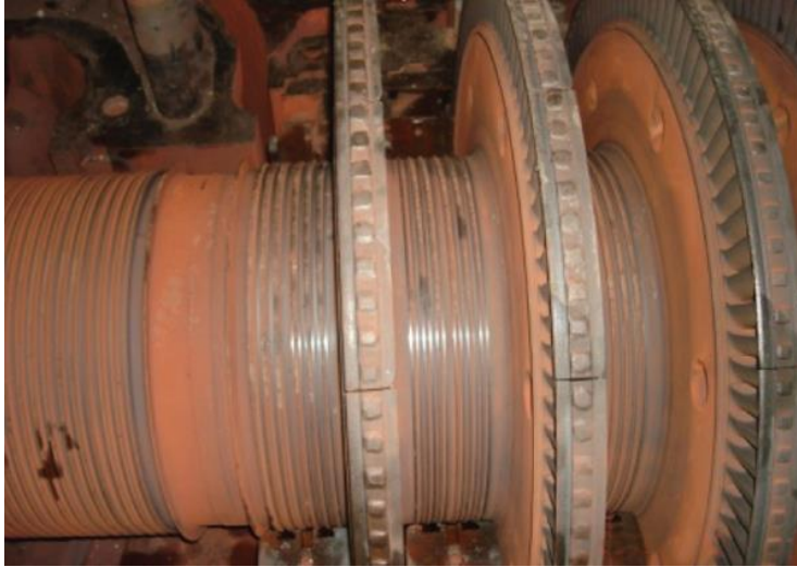
Fig. 3-b Blade rubs cause bending. Rubbing in the sealing of a high-pressure rotor caused bending of this rotor and blade tip rubs. Source: Photo taken at Jordan Petroleum Refinery (2017).
