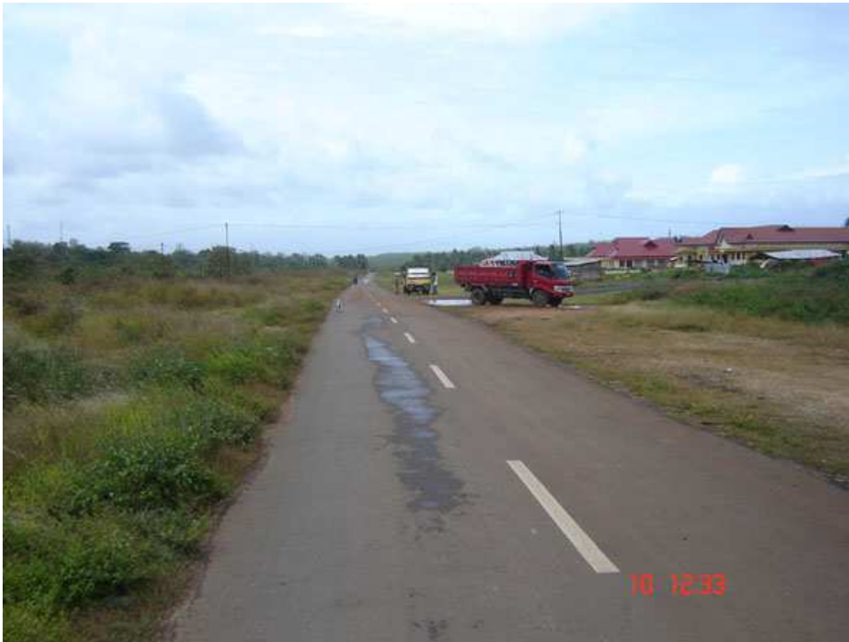
Figure 9 Main road project in Saumlaki town
