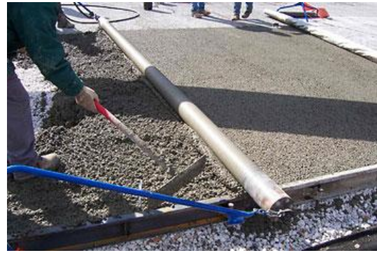
Figure 3: Casting pervious concrete in conventional methods.
