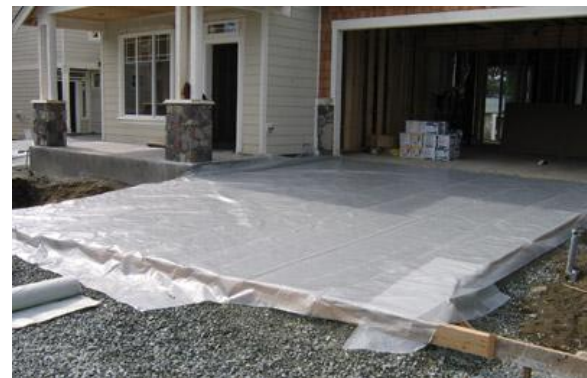
Figure 4: Concrete curing using plastic wrap.
