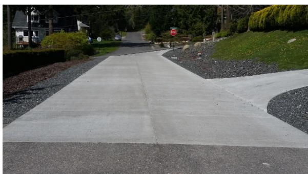
Figure 5: Using pervious concrete in park curb and parking lots.
